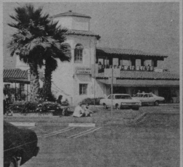
TERMINAL PROBLEMS — The old Santa Barbara air terminal hasn't been able to keep up with increased traffic and local voters will be faced with a bond issue of whether a new terminal should be constructed or an addition put on the present one.
