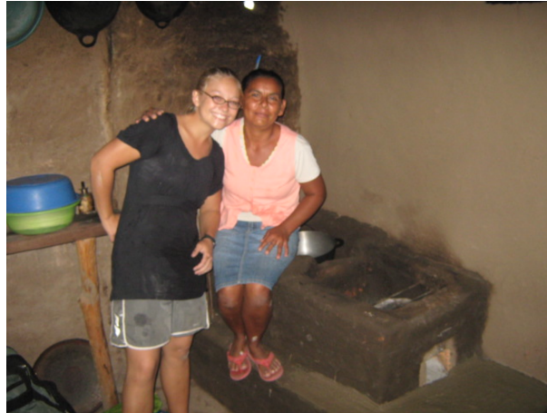
Figure 3. The author and Doña Alina during the construction of her improved stove (2011)
