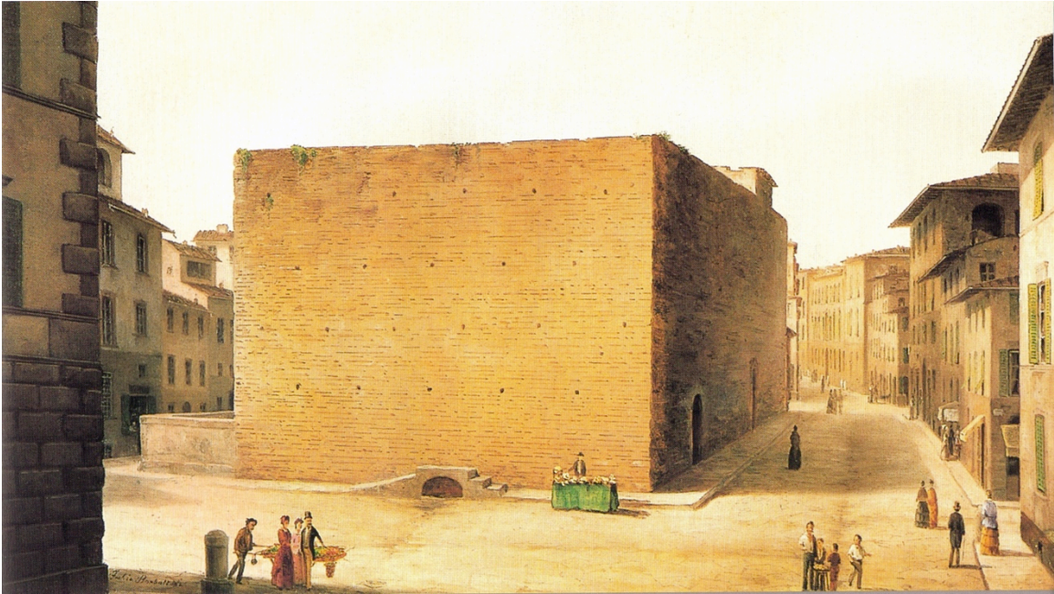
Figure 5: The Florentine public prison, Le Stinche , on the present-day site of the Teatro Verdi. Built on the site of old Uberti properties and named after the Cavalcanti castle at which some early first prisoners were taken, the prison opened in 1302. Oil painting by Fabio Borbottoni, Isola delle Stinche e via del Fosso dal lato di levante from his Vedute di Firenze antica (1820-1902).
