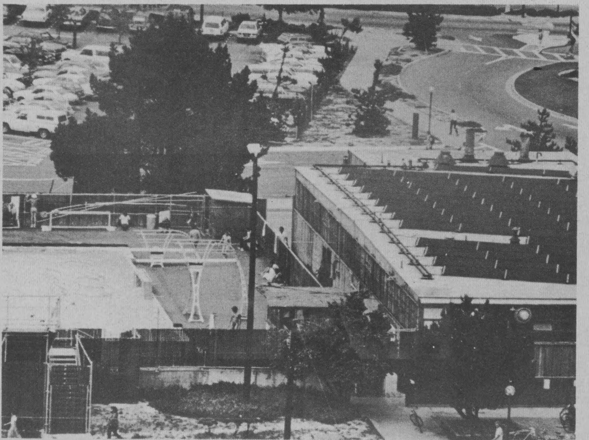
Santa Barbara has long been at the center of this country's environmental movement. The two gentlemen shown at left helped to make Santa Barbara the leader in per-capita conservation efforts. Above, the UCSB Old Gym is bedecked with solar panels that provide most of the heat for the Campus Pool.
