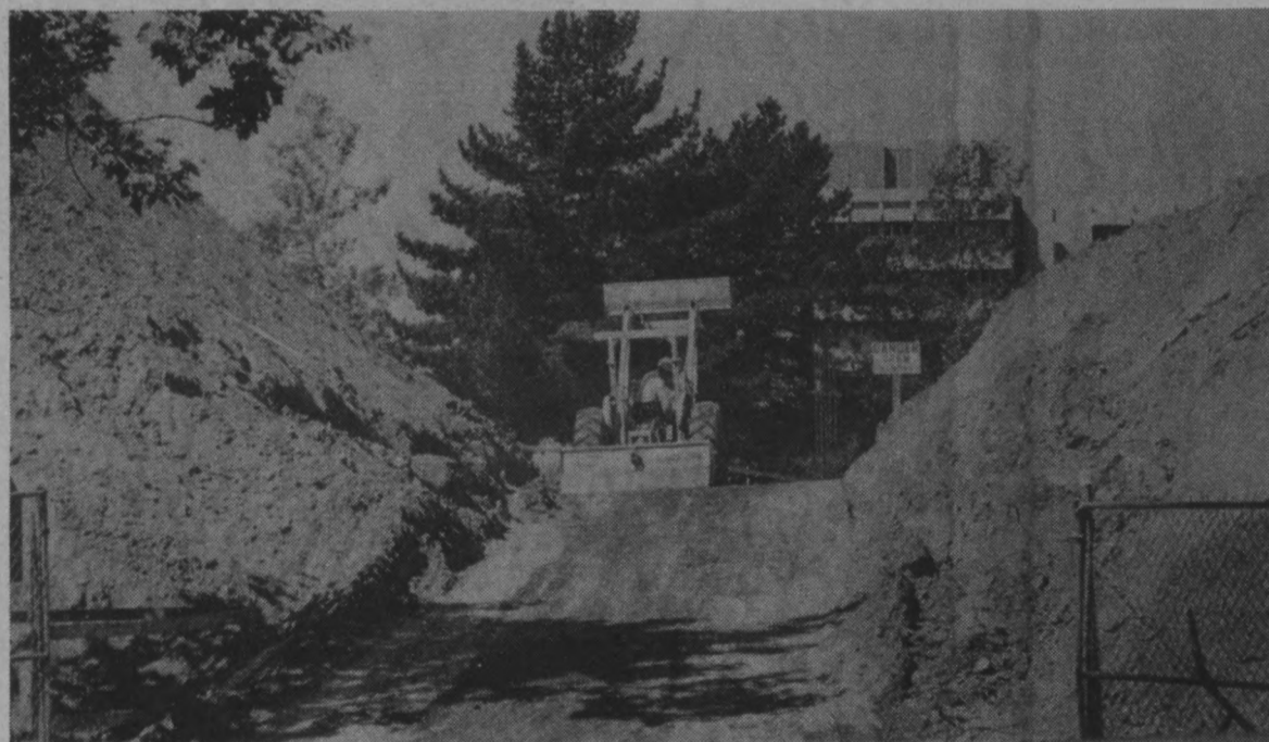
EXPANSION SITE — Controversy has cooled in the building of a new library wing.
