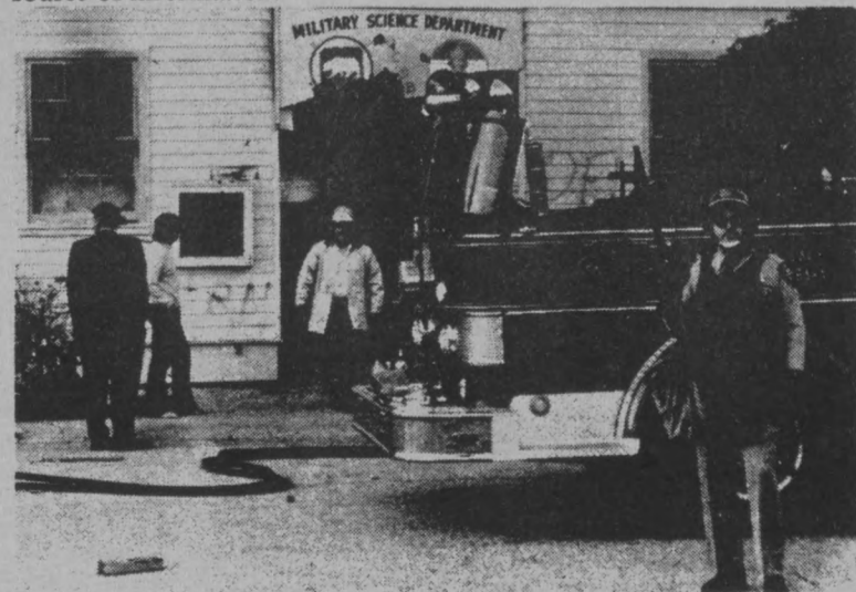
Damaged ROTC building
