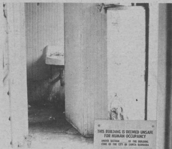
INDOOR PLUMBING—a rarity in Santa Barbara slum housing. —photo by Nelson
