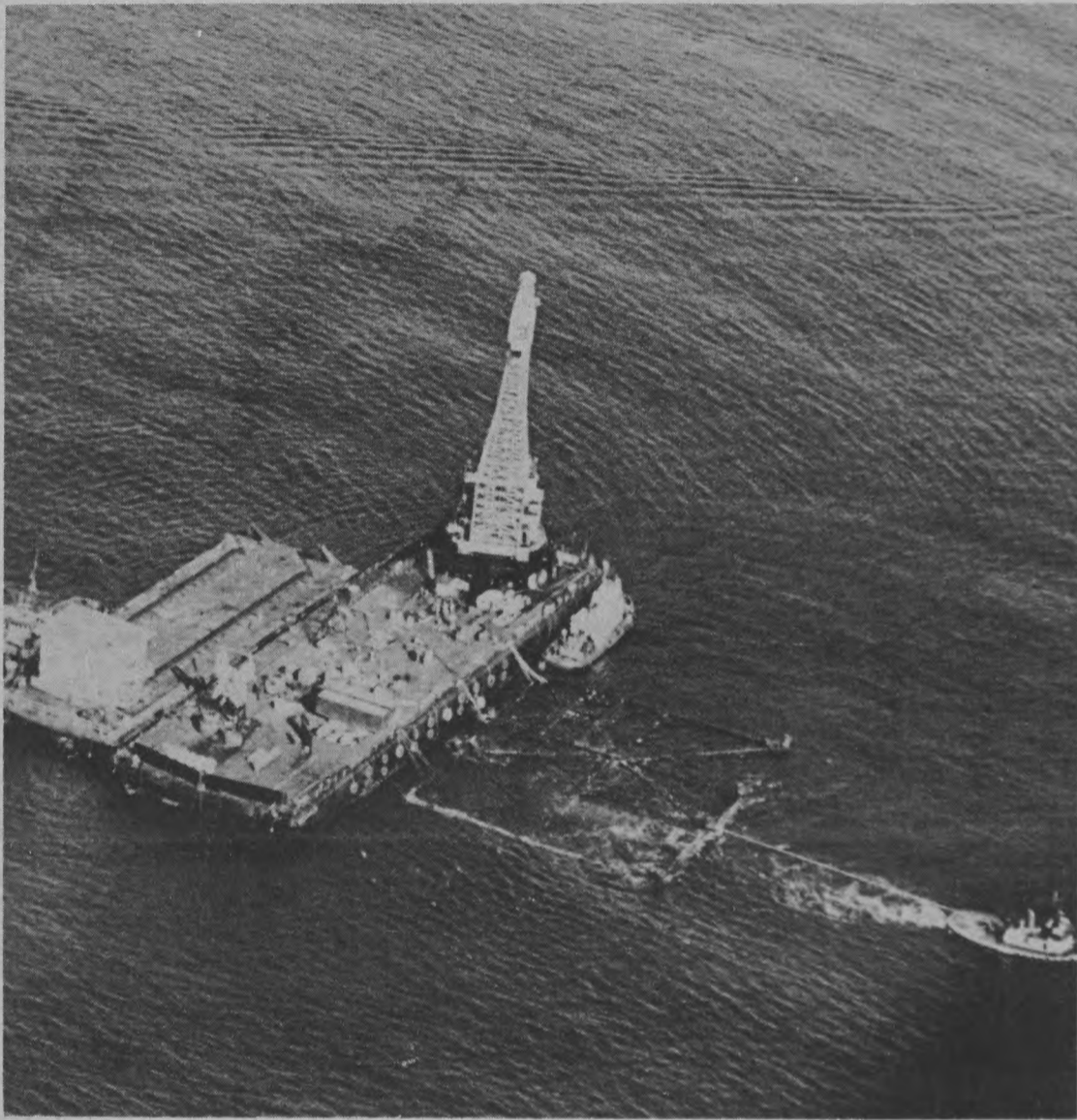
SUN OIL COMPANY'S platform Hillhouse as it floated bottom up two days ago. It is secured to the huge crane barge, William Denny, while the tugboat Donna Foss keeps a taut hawser on the rig. The platform sank later. Photo by Tim James
