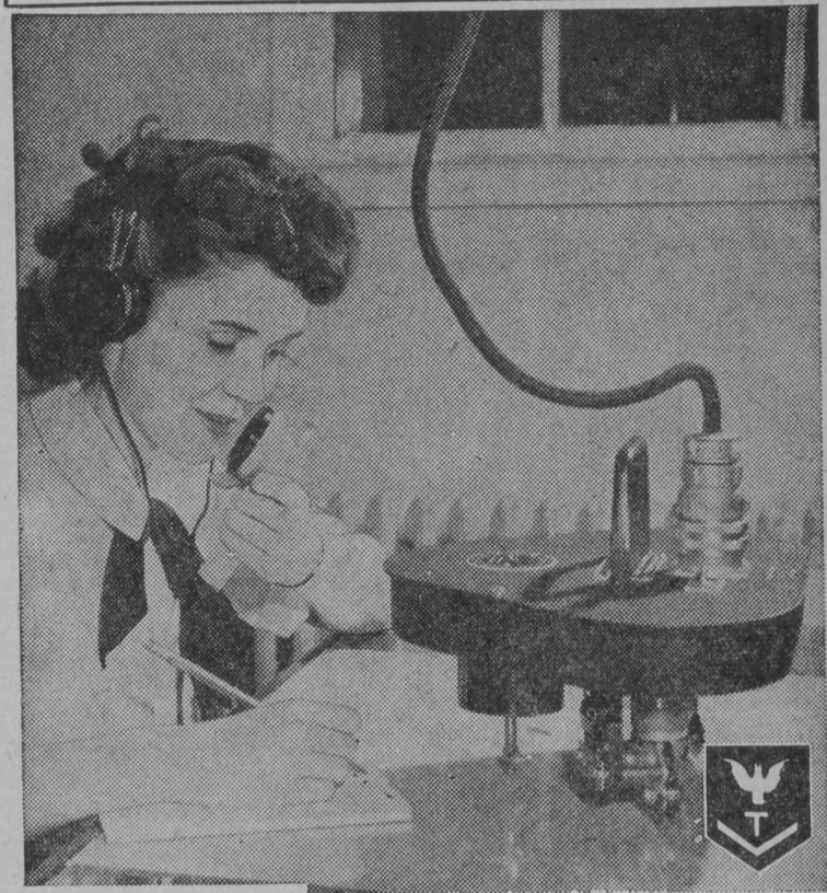
This WAVE—and hundreds like her—helps keep 'em flying. She's an important cog in the machinery which makes Navy fliers. As a Link Trainer Instructor, her job is to give directions to fliers, seated in cockpits of stationary training planes. The instrument in front of her, called a "crab," records how well the pilot carries out those directions. As a result of this kind of training, hazards are greatly reduced for pilots when they go aloft. The inset shows a rating badge worn by Link Trainer Instructors, the "T" meaning teacher. A new booklet about the WAVES is available at Navy Recruiting Offices.
