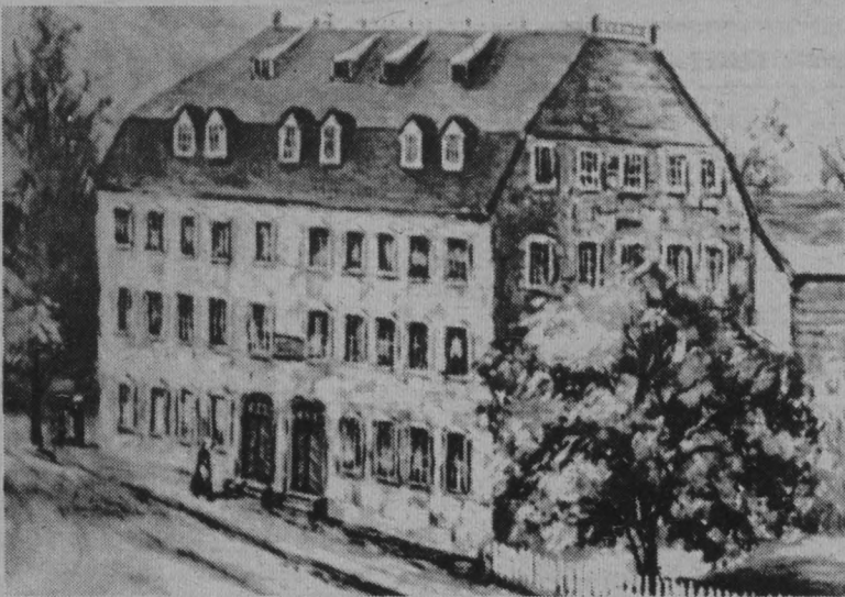
BUILT IN 1748 —When "his Excellency General George Washington" ordered the General Hospital of the Continental Army to be moved to Bethlehem, Pa., this structure, the Single Brethren's House of the Moravian settlement, was converted into a hospital to care for the wounded, who were fed and nursed by the Moravians. These pacifistic and industrious people are among the settlers dealt with by Dr. Robert H. Billigmeier in his new book, "Americans from Germany: A Study in Cultural Diversity."
