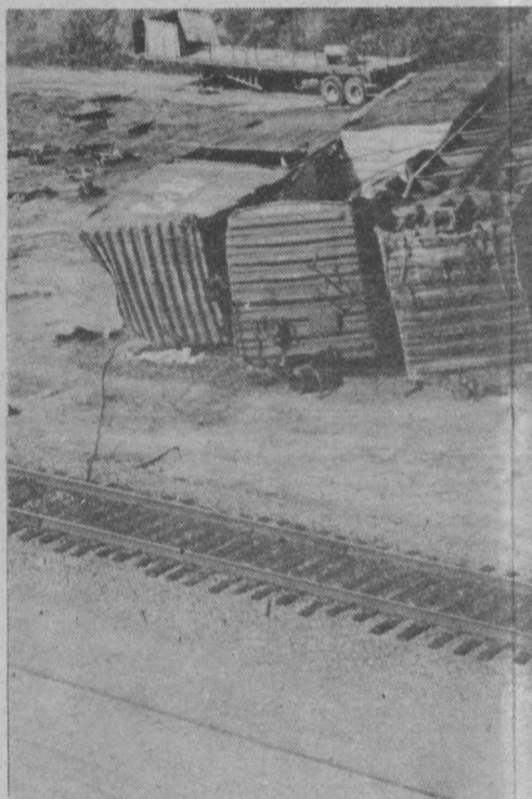
These crumpled train cars were victims of last year's earthquake, and three months ago they were still laying at the exact site of Sunday's incident.
