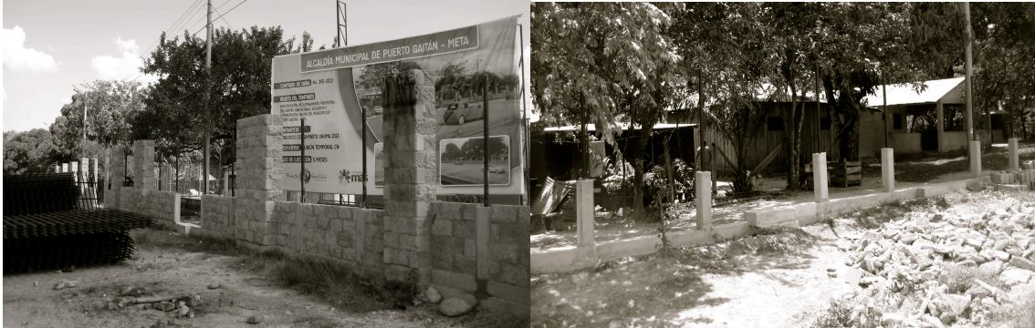
Figure 18. Wall Under Construction Surrounding Siquani Reserve, 2013
