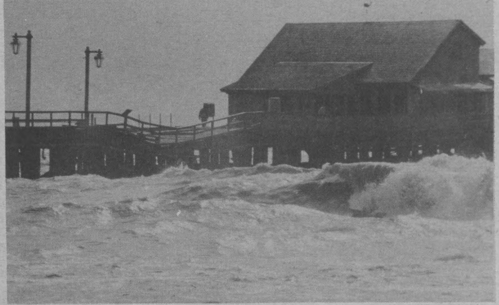
Dick's Restaurant in the drink (right) as pilings were washed away from beneath Stearn's Wharf.
