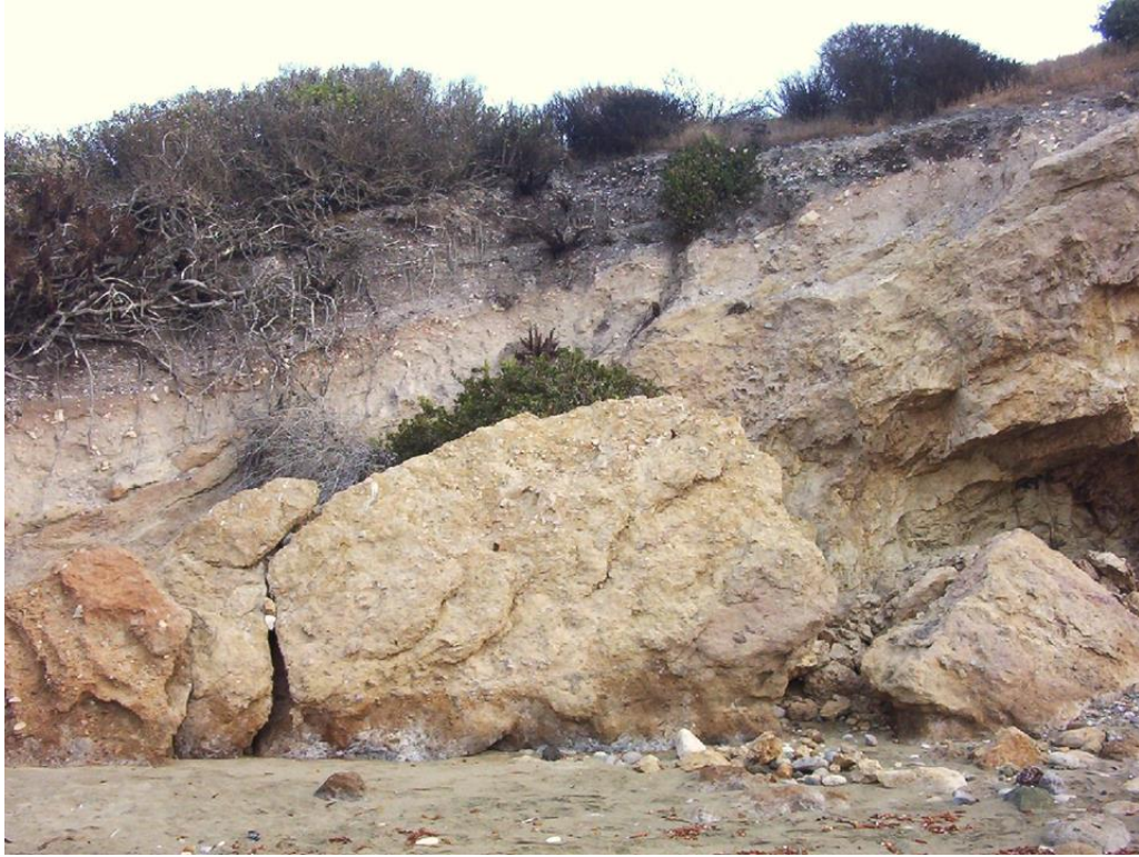
Figure 3. SCRI-496 at Willows. Shell midden resting on the eroding rocky wall.
