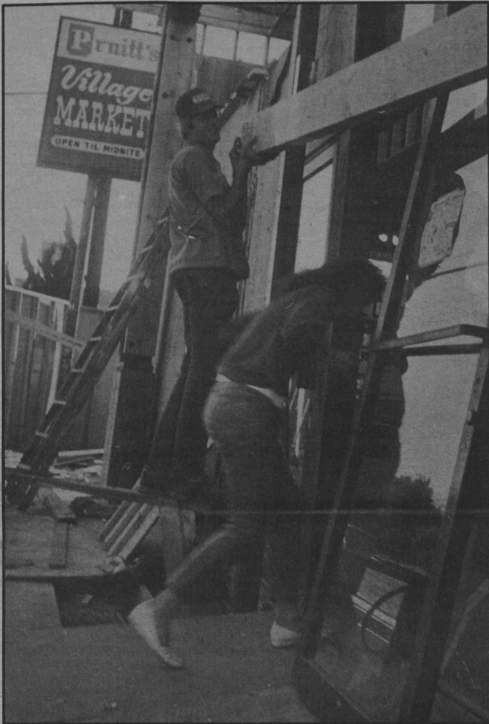
Business As Usual? — Construction work at Pruitt's Market offers the I.V. shopper new challenges daily. This one's called the tuck and dash.
