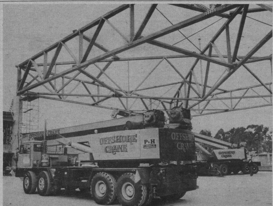
Construction on UCSB's new Events Facility moved one step closer to completion yesterday as this "Offshore Crane" lifted roof beams on to four concrete pillars. (Photo by Karl Mondon)
