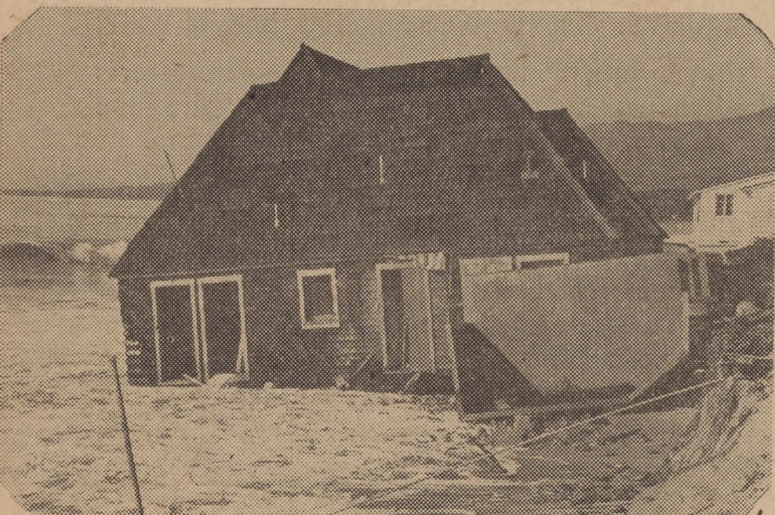
The H. K. Alson, Jr. cottage in Sandylan pictured shortly after it toppled into the surf during high tides. Picture courtesy News Press.
