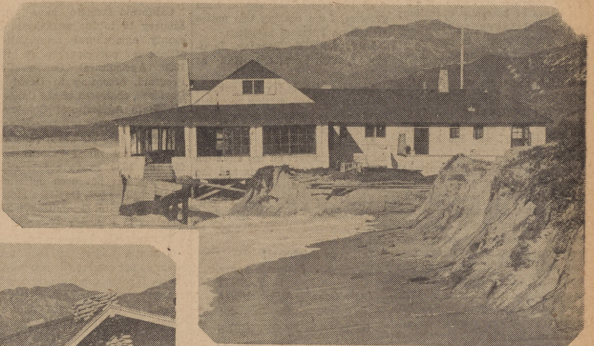
The home of George Owen Knapp, one of the founders of Sandylan, which was seriously damaged but was prevented from collapse by workmen. Picture courtesy News-Press.
