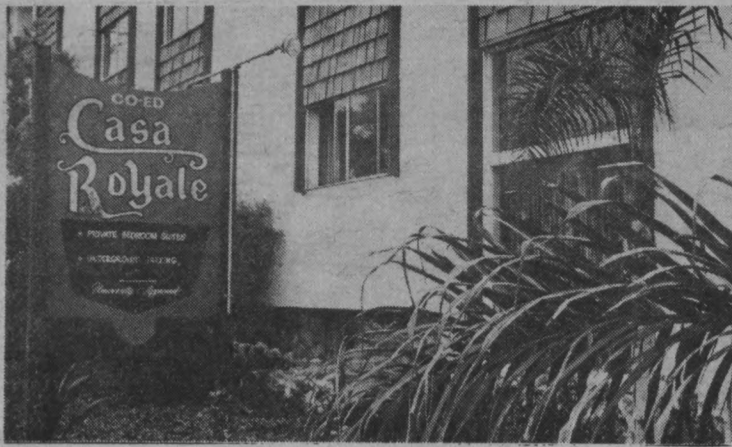
CASA ROYALE'S 156-units will be nearly empty next month when the building closes down for structural repairs and a facelift.
