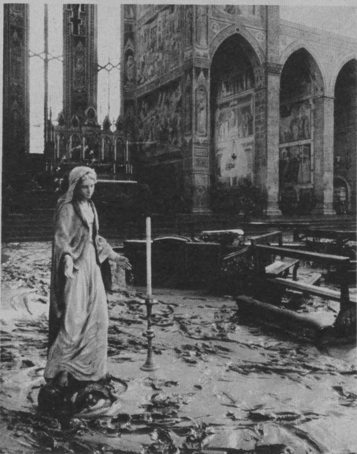
MUD-FILLED Florentine church shows typical flood damage before restoration work began.
