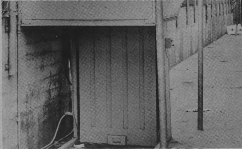
This access to a door on campus in one of UCSB's more outstanding construction projects.
