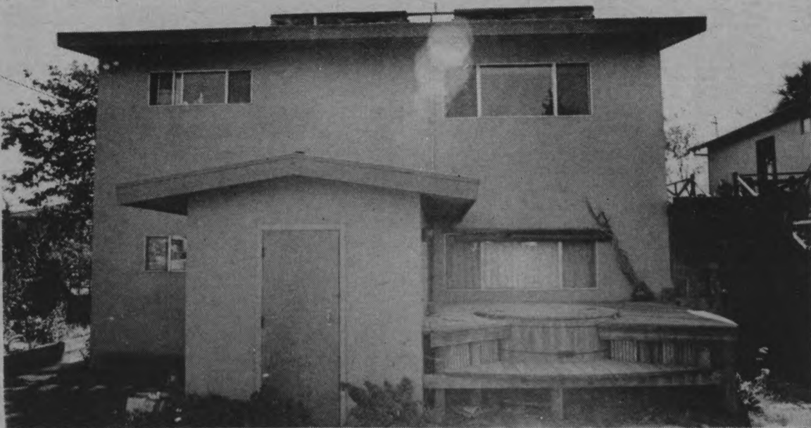
The active solar unit atop this I.V. home provides heat for the hot tub below.
