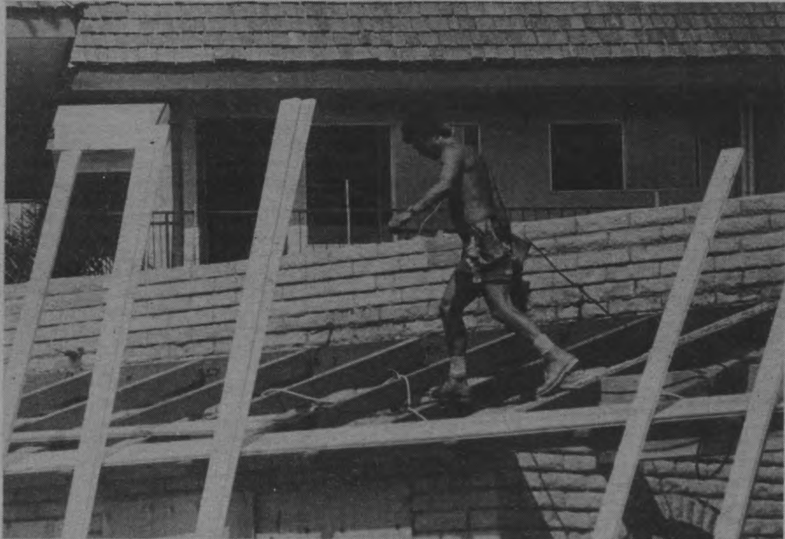
Former Isla Vista Taco Bell under construction.
