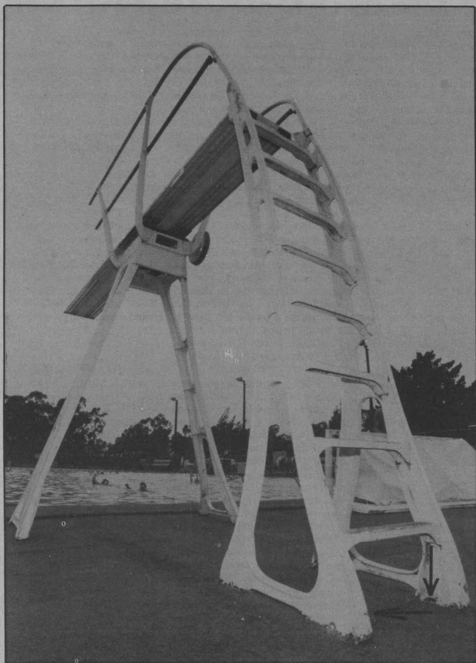
READY FOR PASTURE? — Some bolts holding UCSB's three-meter springboard (arrows) down came loose over the summer. Now a proposal has been put into action by diving coach Mike Lewis to seek out the funding needed to buy a new one.
