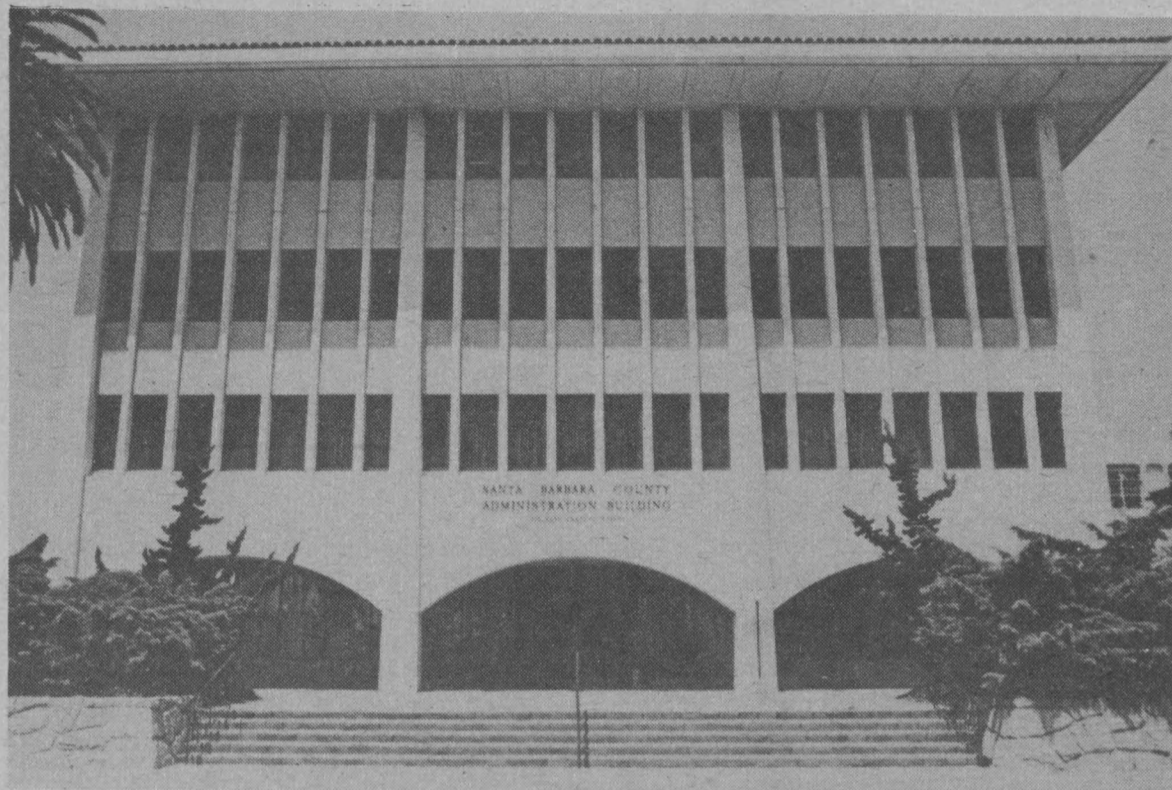
WHERE THE ACTION IS - The Santa Barbara County Administration building houses the various county departments that see to it that the county operates efficiently on a day to day basis.
