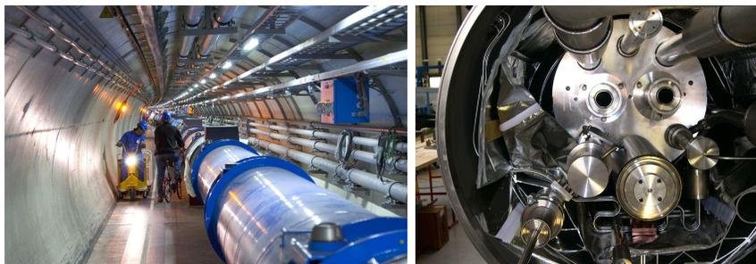
Figure 3.2: Photographs of the LHC. A view of the accelerator inside the underground tunnel (left), and a cross-sectional view of a dipole magnet (right). Photos: CERN.
