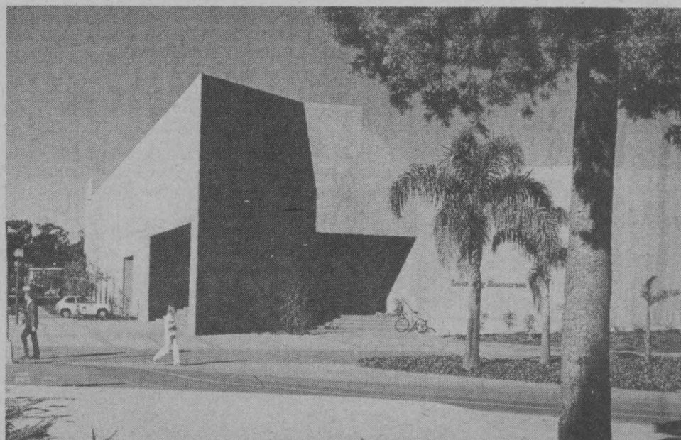
LEARNING RESOURCES – UCSB's newest addition to the campus which offers facilities to improve all levels of teaching and communication will be dedicated at 10:30 a.m. on University Day.
