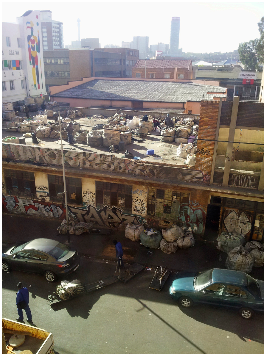
Figure 13. Recyclers' Building, Fox Street. Source: Author's Photograph, 2014.
