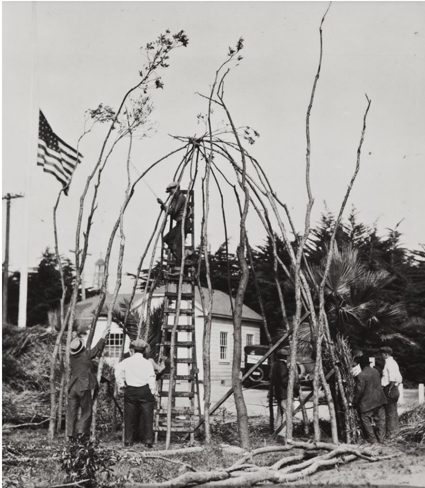
Figure 5.2. Reconstruction of a Chumash house for the 1924 Ventura County Fair. John P. Harrington oversaw the project, and the structure was built by Chumash men, including José Winai, who was one of Harrington’s Ventureño Chumash consultants. Smithsonian Institution: J. P. Harrington Collection. Courtesy of the University of California’s California Digital Library. Contributed by Black Gold Cooperative Library System.
