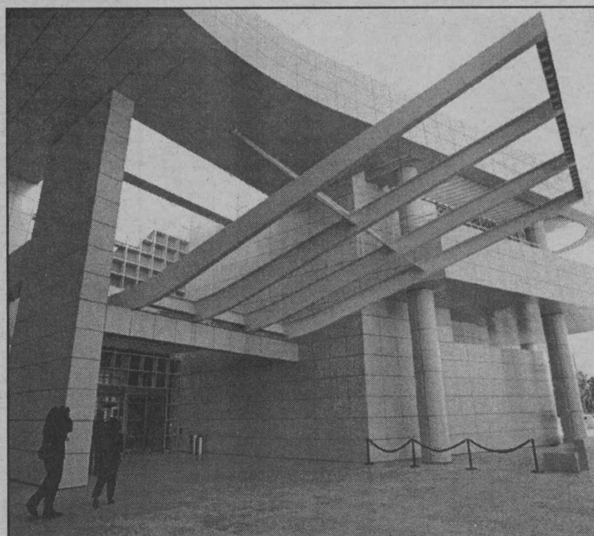
The Getty Museum Entrance Hall, shaped in the manner of a modernist temple, masks its grand interior circular space. Meier's play of geometric forms and materials draws visitors naturally inward.
