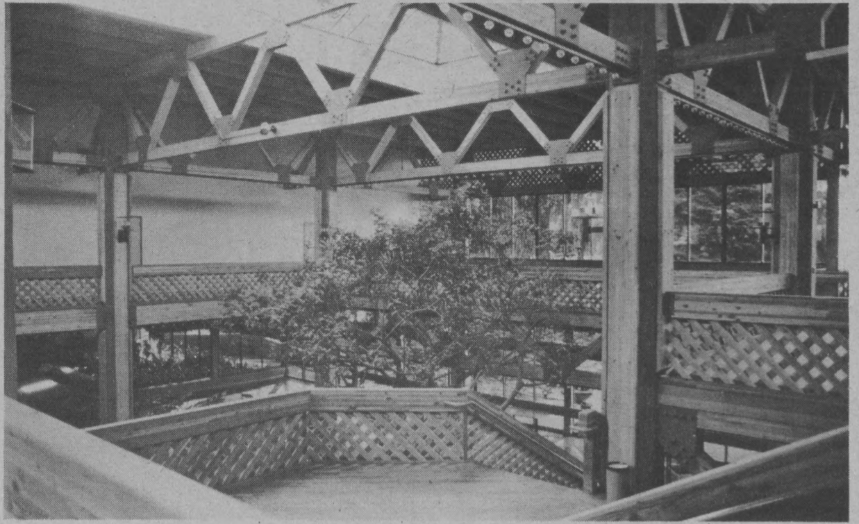
The final touches are now being done on UCen II after nearly two years of construction delays and other problems (see story below).
