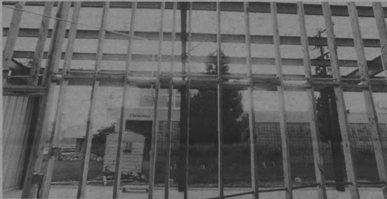
Construction of Engineering II has displaced campus parking spaces.
