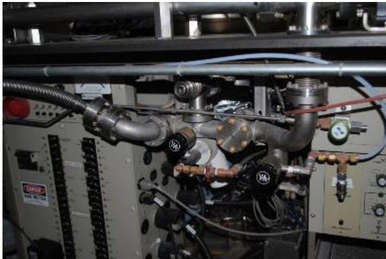
Figure 7 -- External portion of the system manifold showing the gas inlets as well as the connection to the main chamber's metal seal valve.
